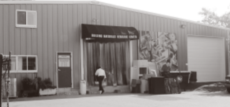
The new addition on the right, with its closed overhead door, blends in seamlessly with the existing warehouse building.
