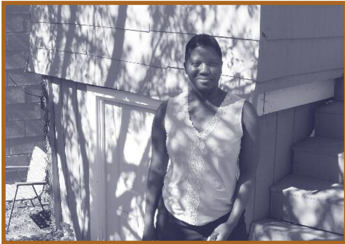
The siding of Linda's home, which had been damaged by an automobile, was repaired by a contractor from the Co-op's tradesperson referral file.
