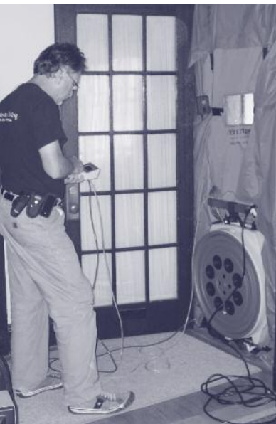
A blower-door test measures the amount of air that flows through a house and allows one to detect areas of air infiltration.
